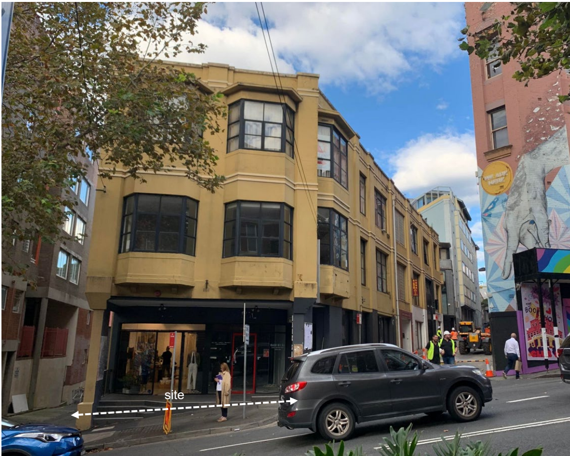
site viewed from Crown Street looking east
