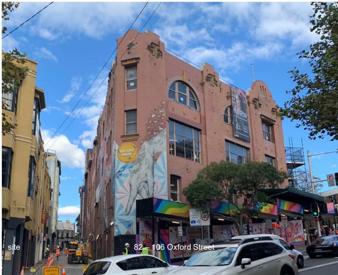
view towards neighbouring building at 82-106 Oxford Street to the south
